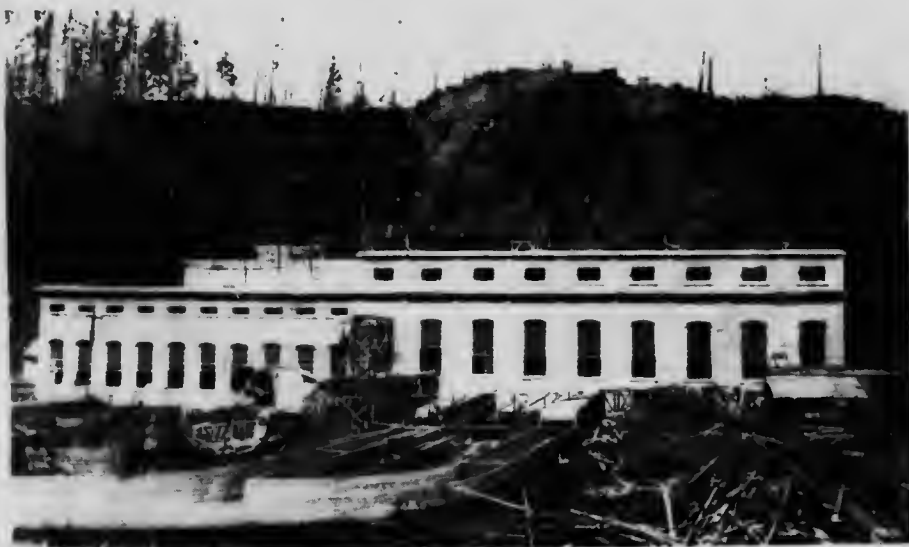
Vancouver Island Power Company Limited. Front view of Power House showing completed building and tailraces.
